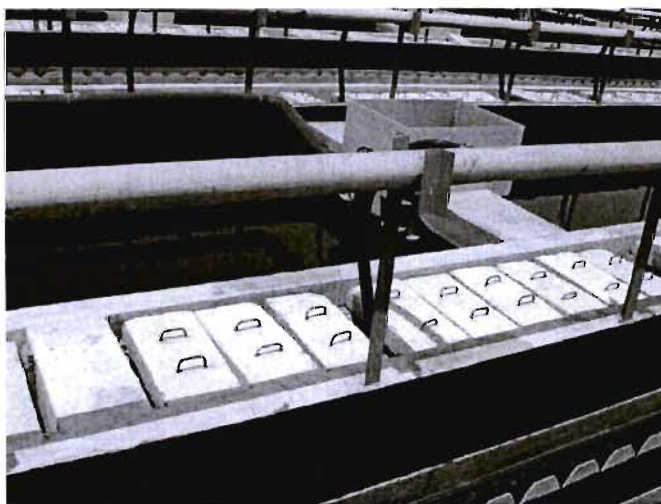
Figure 4-3: UASB with biogas capture (pipes at top) at NWWTP
